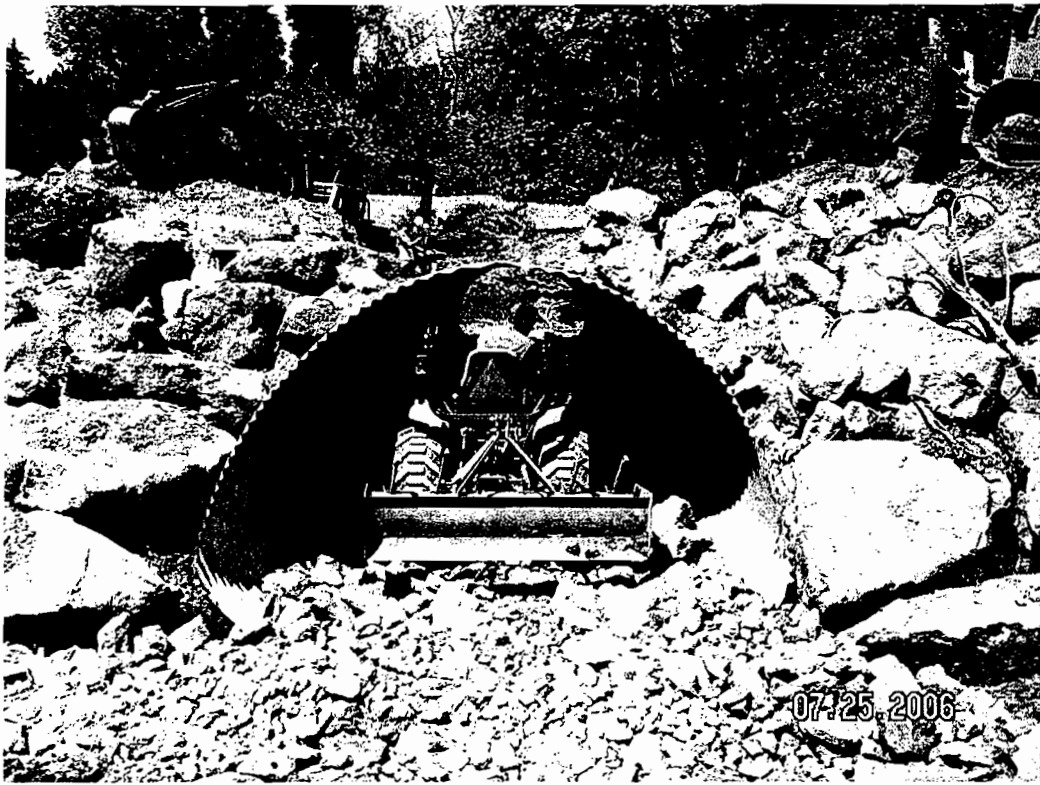
Culvert #1 – Placing the Embedded Rock
