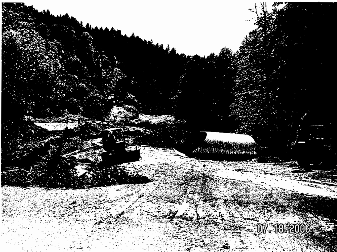
Excavation of Culvert #1
