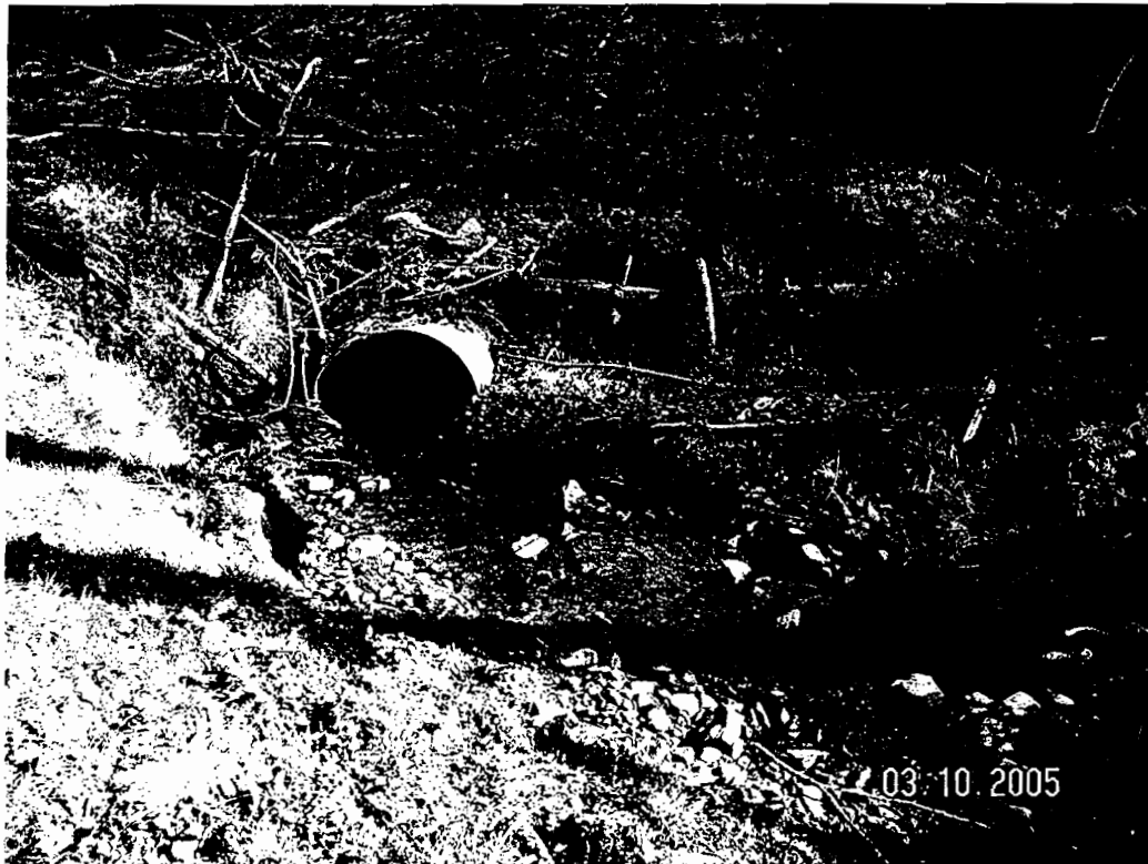
Dodge Canyon Creek – Culvert #2 (March 2005)
