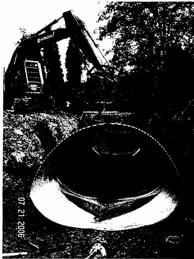
Culvert #1 – Bolting the Sections Together
