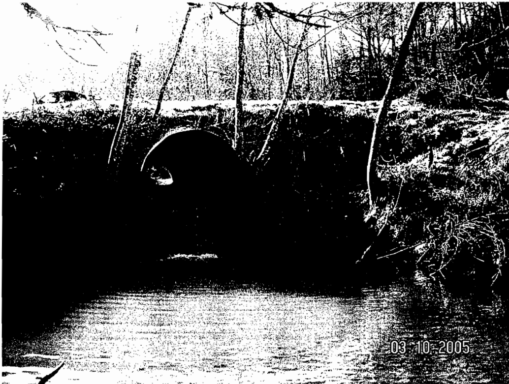
Dodge Canyon Creek – Culvert #1 (March 2005)
