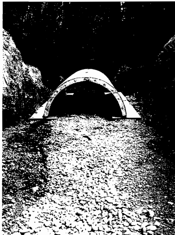
Culvert #3 – First Section on Rock Foundation
